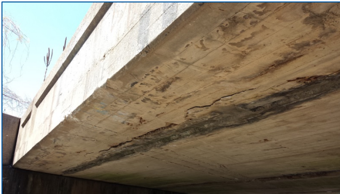
Concrete damage to the underside of the superstructure
